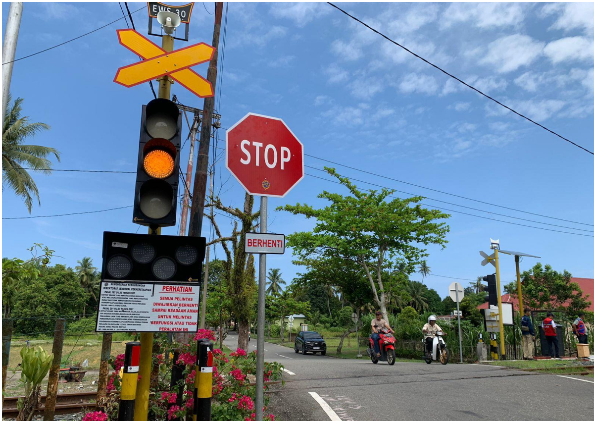
Figure 1. Early Warning System (Class II Padang Railway Engineering Center, 2023).
