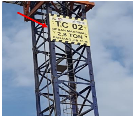
Gambar 3. Rambu beban maksimal tower crane
