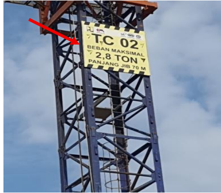
Gambar 3. Rambu beban maksimal tower crane
